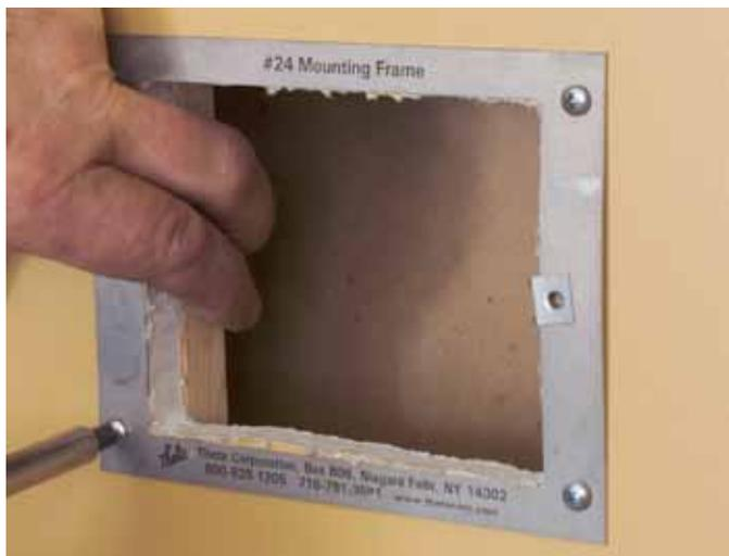
Installing wood scrap behind drywall for #24 Mounting Frame
