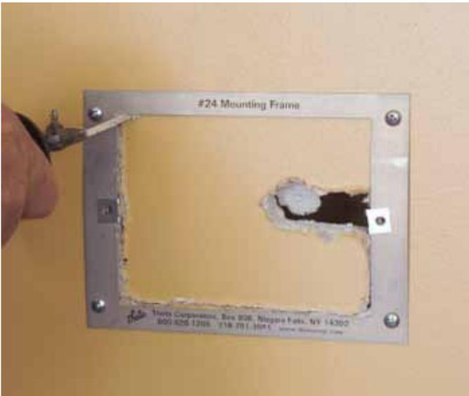
Sawing out hole in drywall behind #24 Mounting Frame
