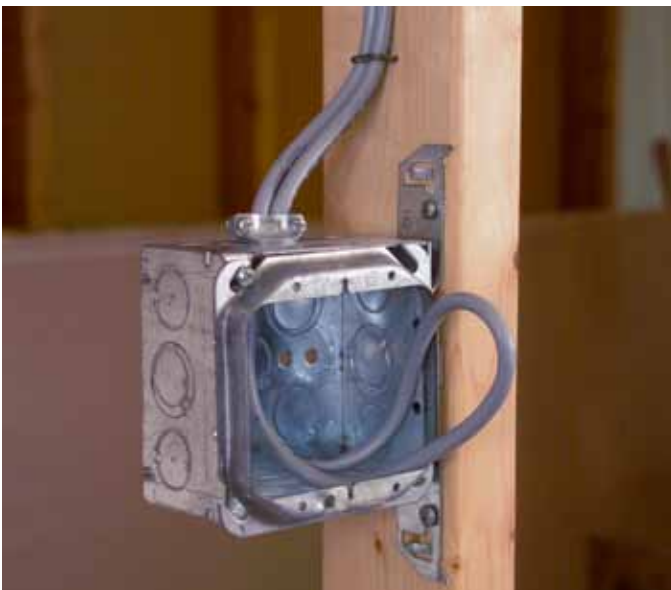
4" Square Box with Two Gang Reducing collar
